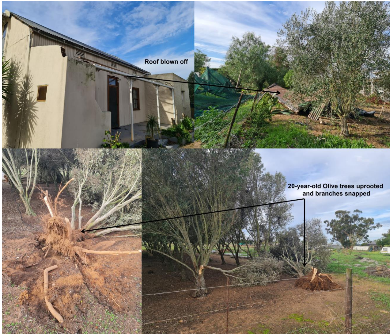
Figure 1: Evidence of the damage caused by the landspout. The top photos are of a roof that was blown off and the bottom photos of 20-year-old Olive trees that were uprooted, and branches snapped.
