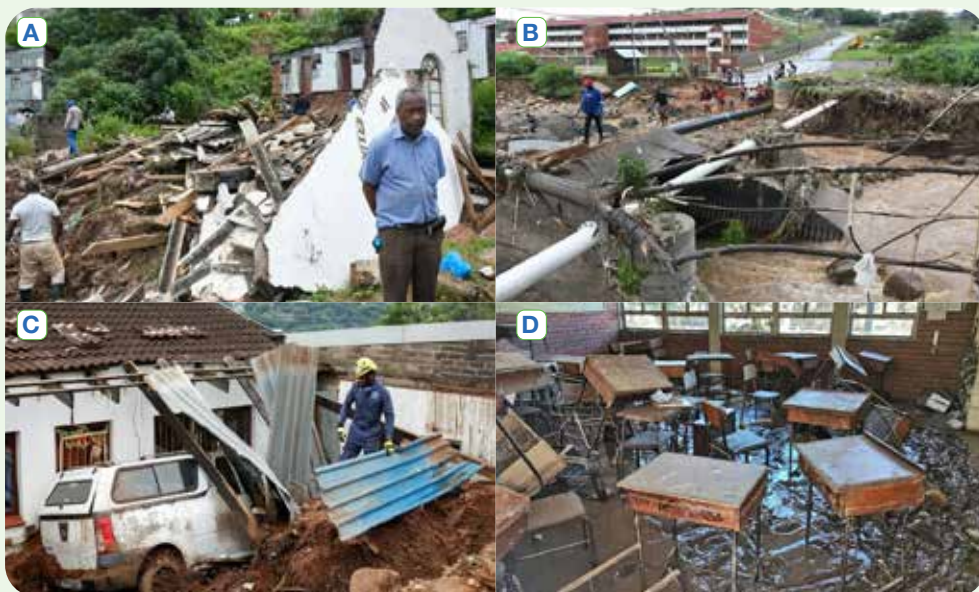
Photographs: A and C indicate damage to houses in parts of KwaZulu-Natal (Source: BBC News). B showing damage to road and bridge infrastructure (Source: Flood list). D indicating a flooded school classroom (Source: UNICAF SA)
